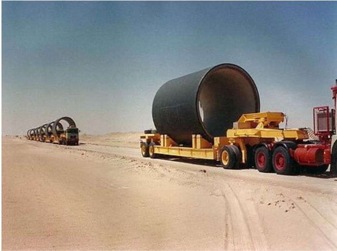
**Fig, 26.** Transportation of pipe segments in the 1980s for the Great Manmade River in the Sahara Desert, Libya. This network of pipes supplies water from the Nubian Sandstone Aquifer System, a fossil aquifer in region. The Great Manmade River is the world's largest irrigation project with abstraction estimated at 2.4 km<sup>3</sup> per year. With many thanks to Jaap Berk.
